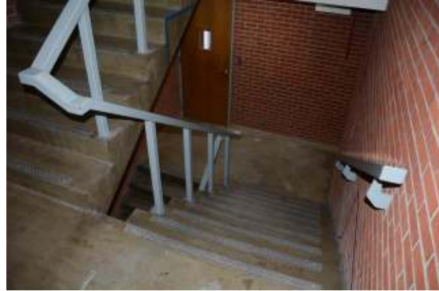
Non-accessibility code compliant restrooms, stairwell railings. Though some compliant features have been introduced, these non-compliant conditions are found throughout the building.
