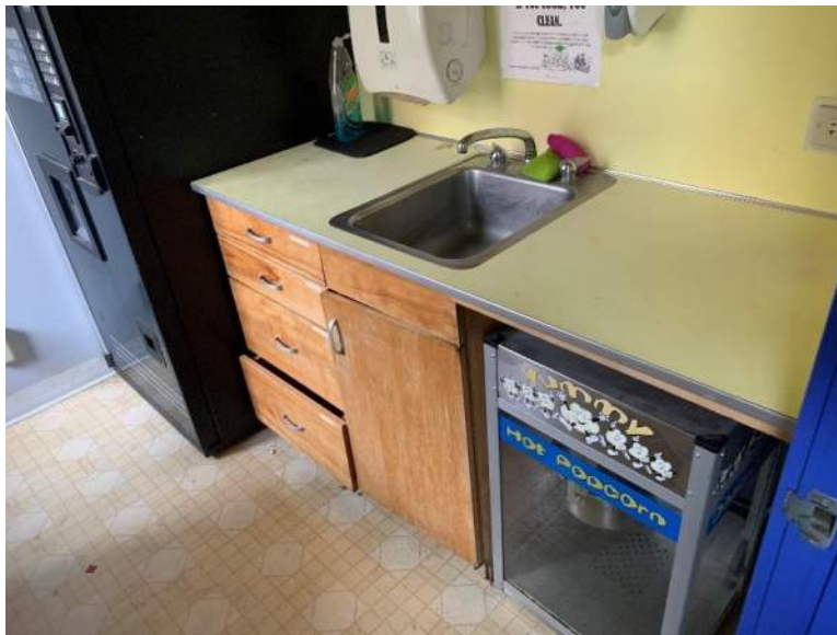
Photo 17: Student Center kitchenette slated for remodel
