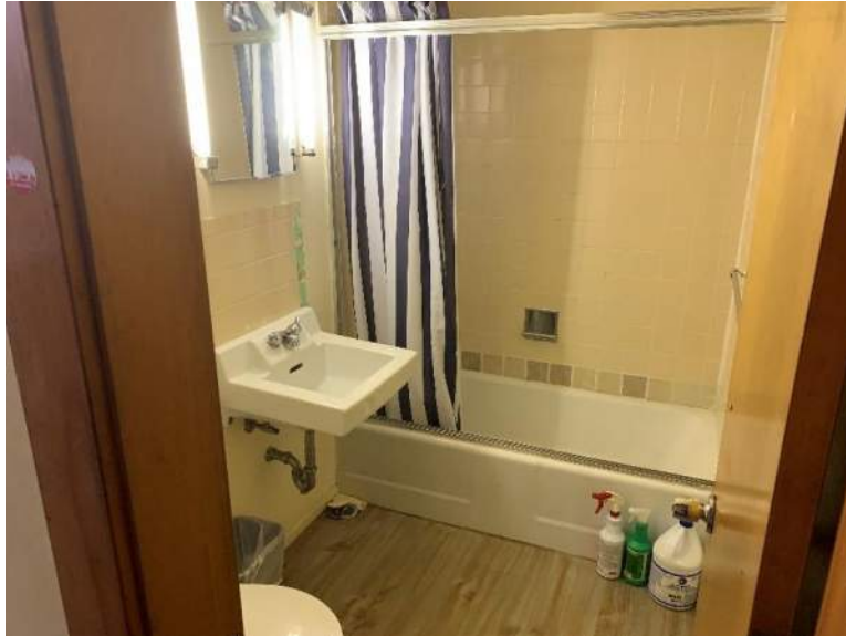
Photo 19: Student Center apartment restroom
