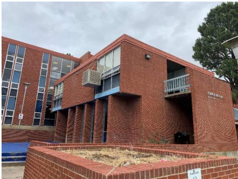
Photo 56: Huggins Hall resident apartment evaporative cooler
