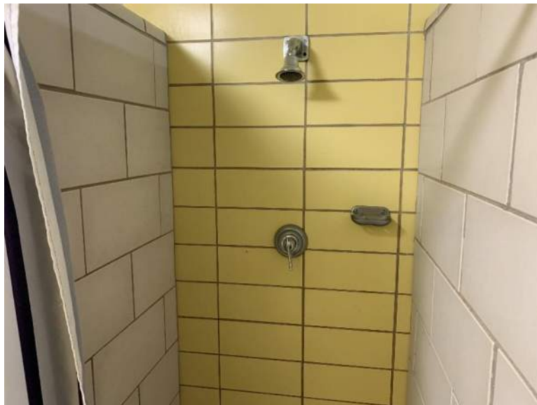
Photo 24: Johnson Dormitory shower stall
