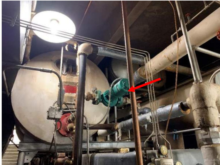
Photo 5: domestic HW storage tank above boiler; potential ACM pipe insulation
