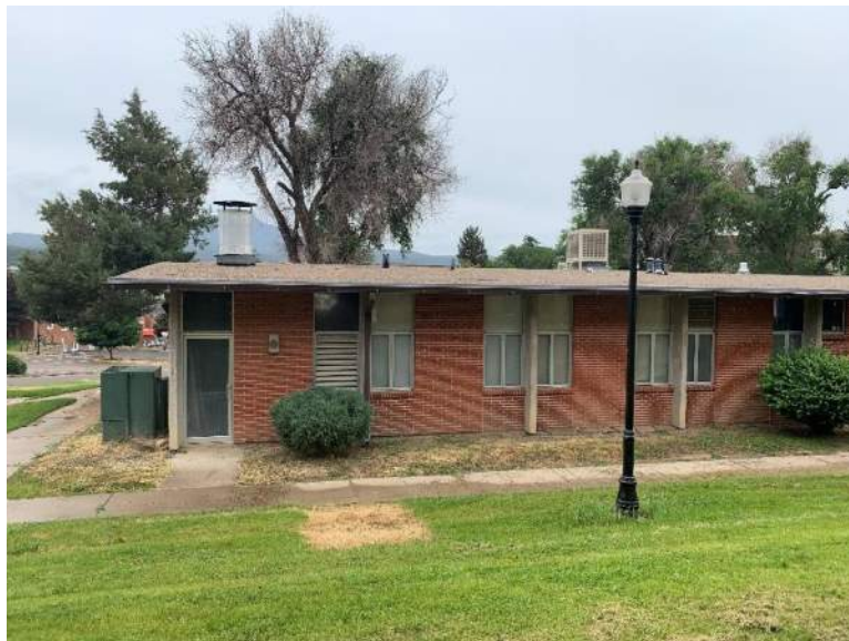
Photo 3: Boiler room entry, combustion air vent, existing boiler flue
