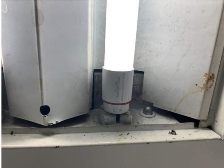
Photo 51: Typical LED fluorescent tube replacement
