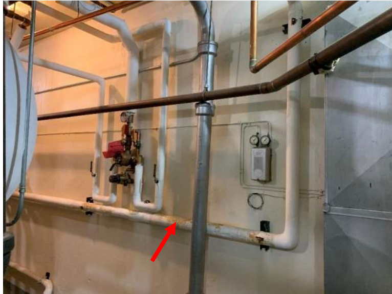
Photo 48: O'Connor thermostatic mixing valve requires connection from recirculated hot water
