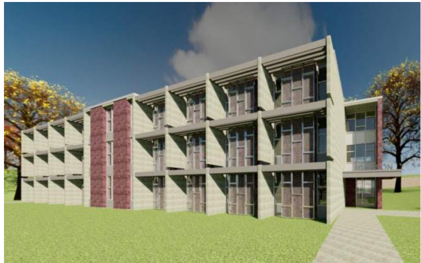
Proposed exterior treatments for Johnson Residence Hall / Romero Residence Hall include metal trellis members anchored to precast panels and wire mesh screen panels to cover select brick surfaces and provide shade to sleeping rooms facing south. Source: Hall Architects.
