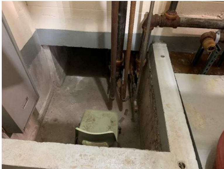
Photo 43: O'Connor boiler room tunnel access
