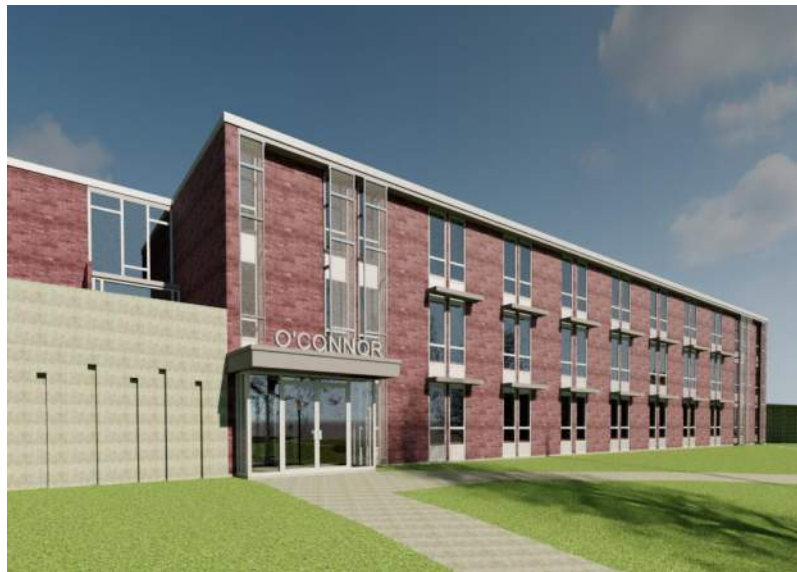
Proposed redesign of O'Connor Residence Hall Pine Street entrance includes repurposing one dorm sleeping room for a welcoming larger entry vestibule with new glass storefront, and a small; ground level student commons area. Provides building with identifiable front door. Source: Hall Architects.
