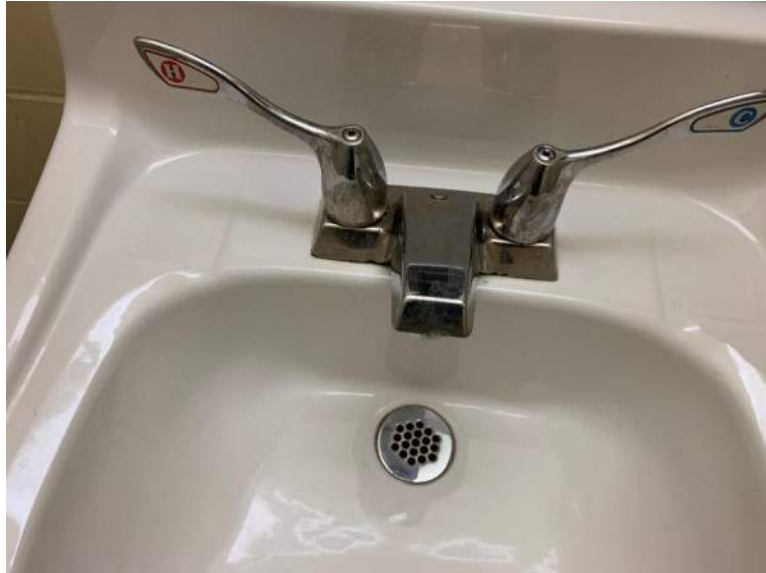
Photo 13: Existing wall hung lavatory with ADA compliant handles
