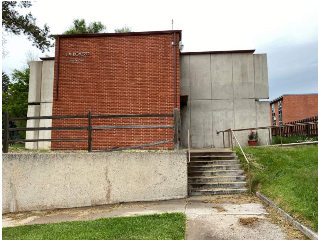
Figure L. Exterior guardrails at Romero Residence Hall entrance. Source: Hall Architects.
