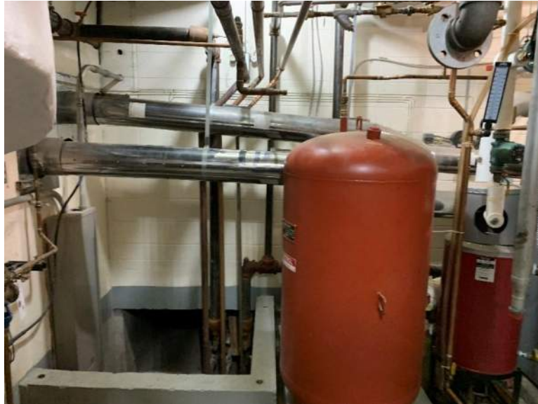
Photo 42: O'Connor boiler room tunnel access
