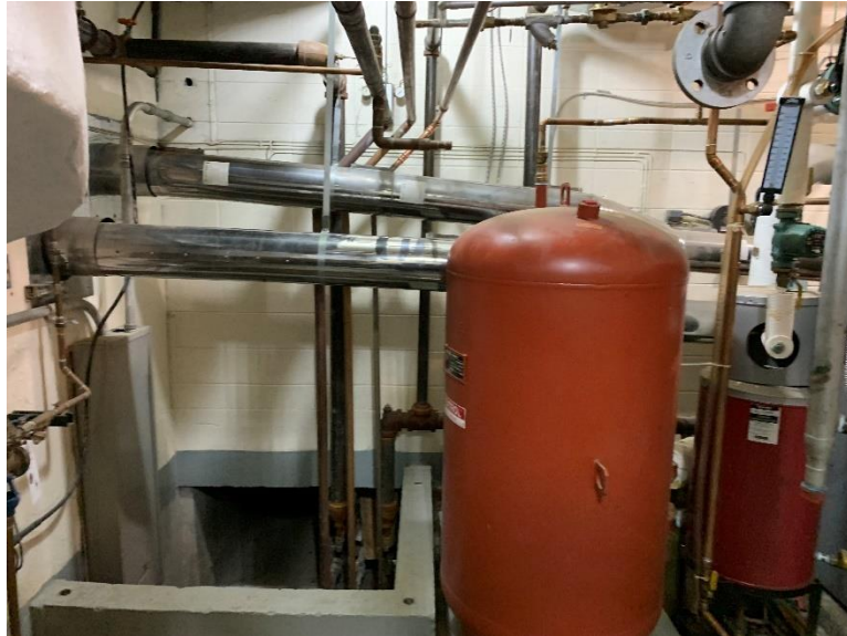
Photo 42: O'Connor boiler room tunnel access
