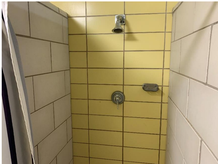
Photo 24: Johnson Dormitory shower stall
