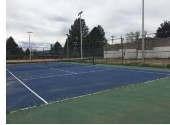
Existing tennis court north of O'Connor.
