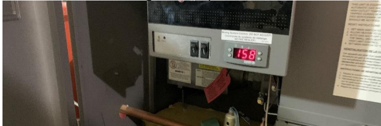
Photo 48: O'Connor thermostatic mixing valve requires connection from recirculated hot water
