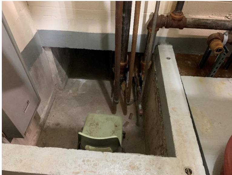
Photo 43: O'Connor boiler room tunnel access
