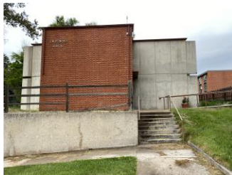
Existing street-facing Romero Residence Hall entrance.
