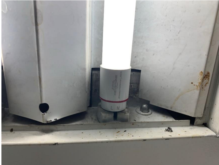
Photo 51: Typical LED fluorescent tube replacement
