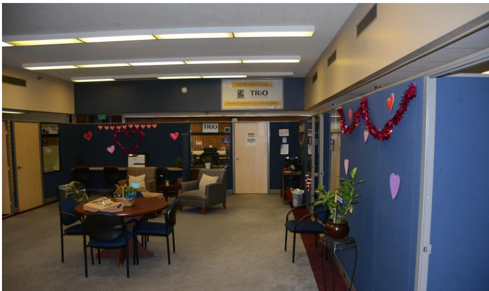
Half height partitions. Shown on the perimeter of these study tables and chairs, these partitions can't control unwanted distracting conversations and noises.
