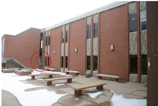
Location of future glass vestibule, noted by red circle.
