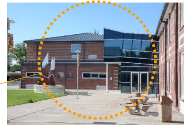
PR1: New Phase 1A Main Building Addition for Student Services “One Stop” at First Floor, Offices at Second Floor
