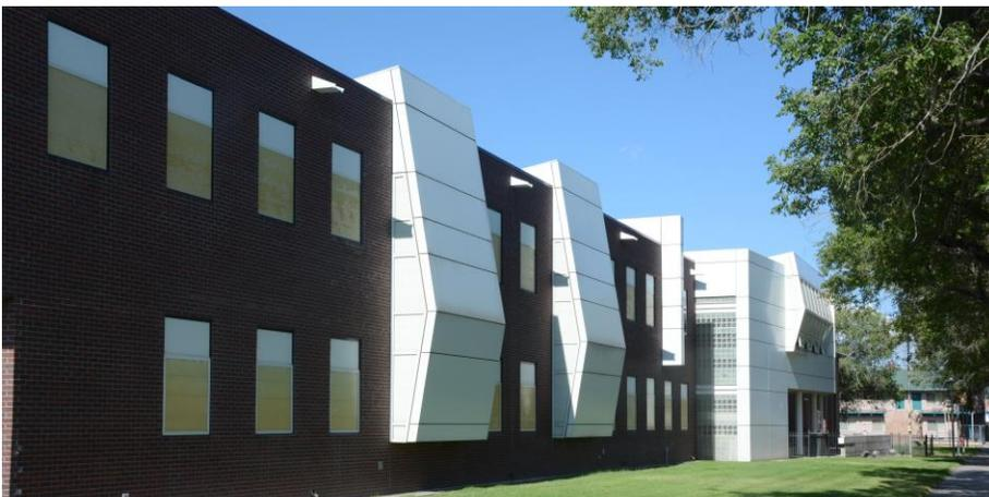
*The plastic of existing windows has degraded and gives the appearance of plywood and the perception of boarded up windows.*
