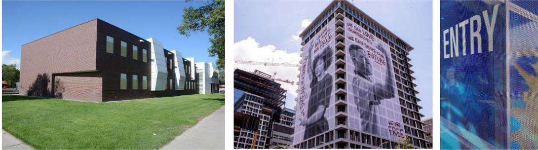
*South elevation of the Main Building (left) with Kalwall glazing planned to receive vinyl wrap material with photo and graphic images (center and right).*
